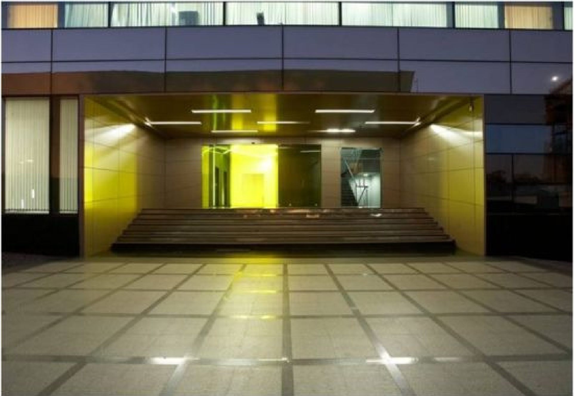
Hi-tech City facility, Hyderabad
